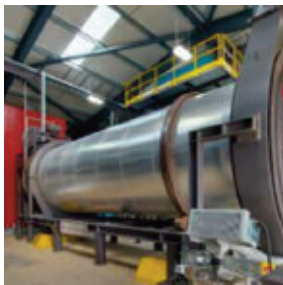
Horizon + the first self-cleaning rotary watertube boiler designed for complex fuels. As courtesy of Sugimat
