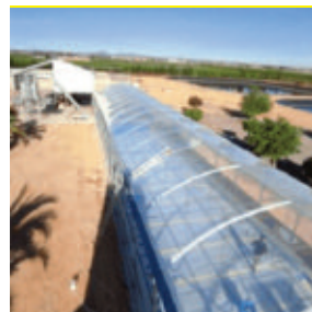
Integration of solar drying and gasification in the valorisation of sewage sludge at a full-scale pilot plant. As courtesy of Ceder-Ciemat
